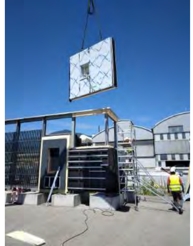
Prefab module with BIST cladding
