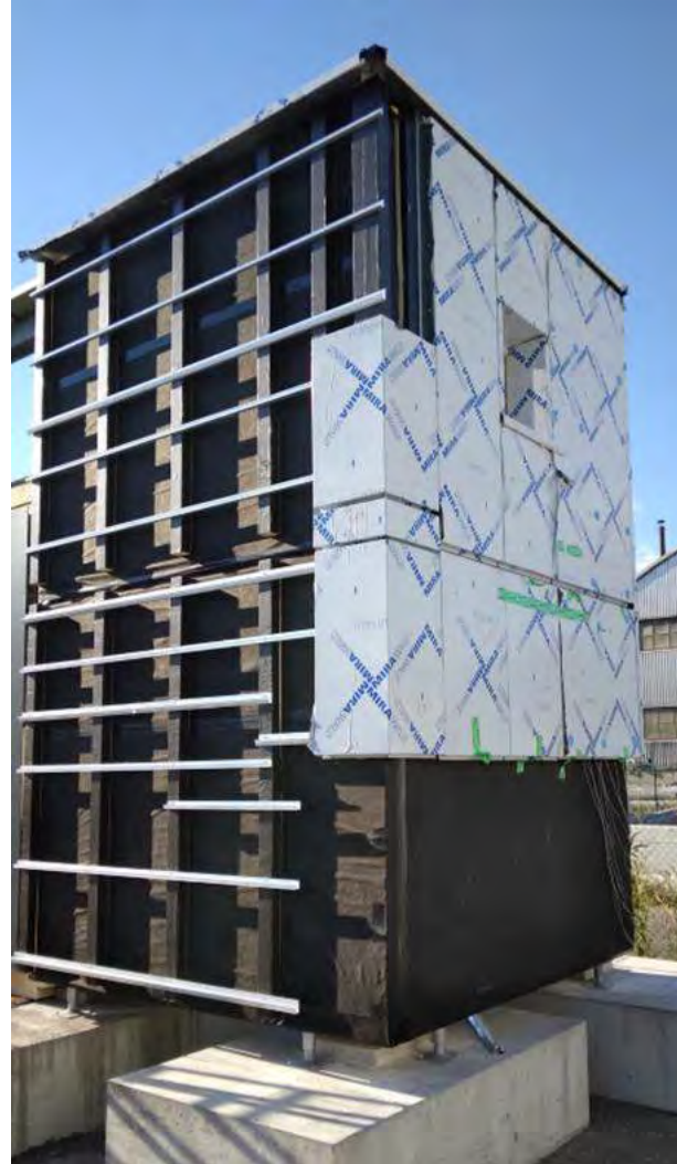
BIST corner installation on-site
