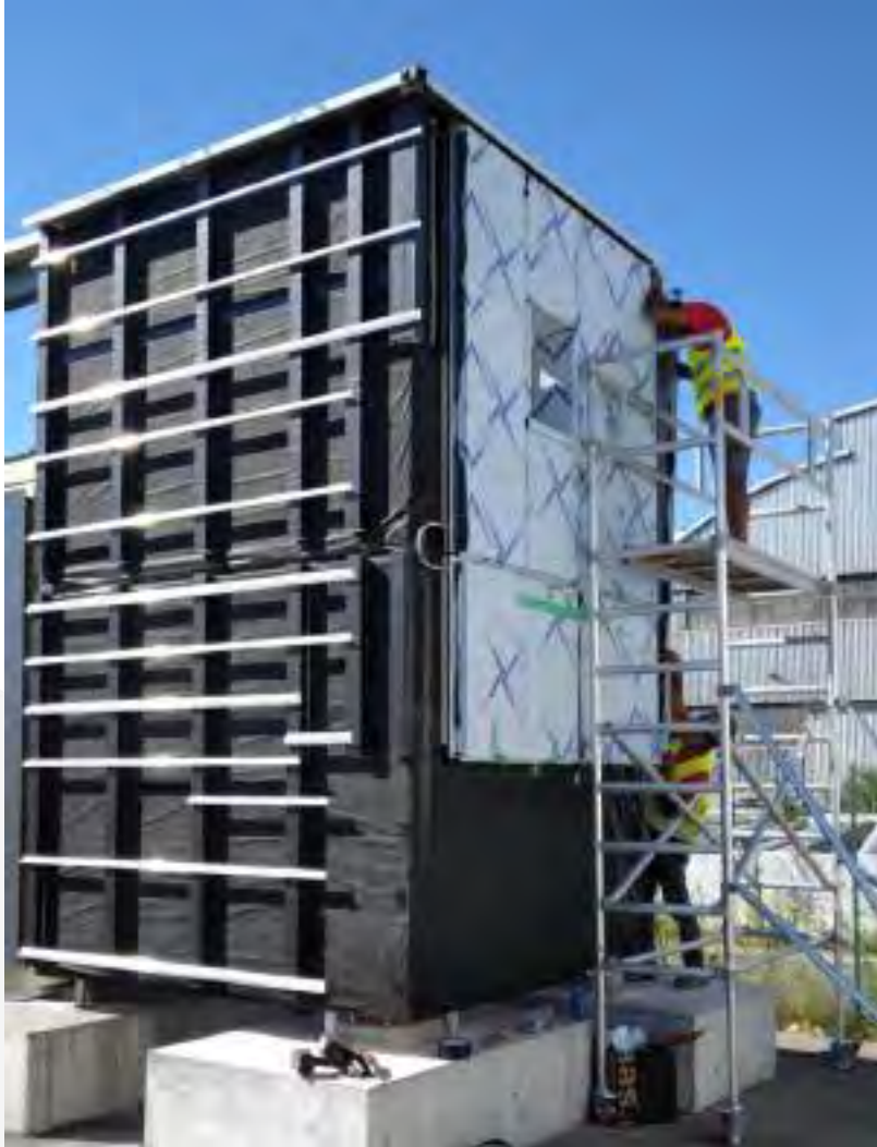
Base structure manufactured offsite
