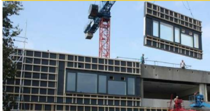
Prefabricated wooden based facade-roof
