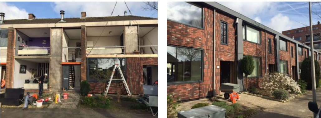
Figure 32 Prefab renovation with total replacement of the façade
