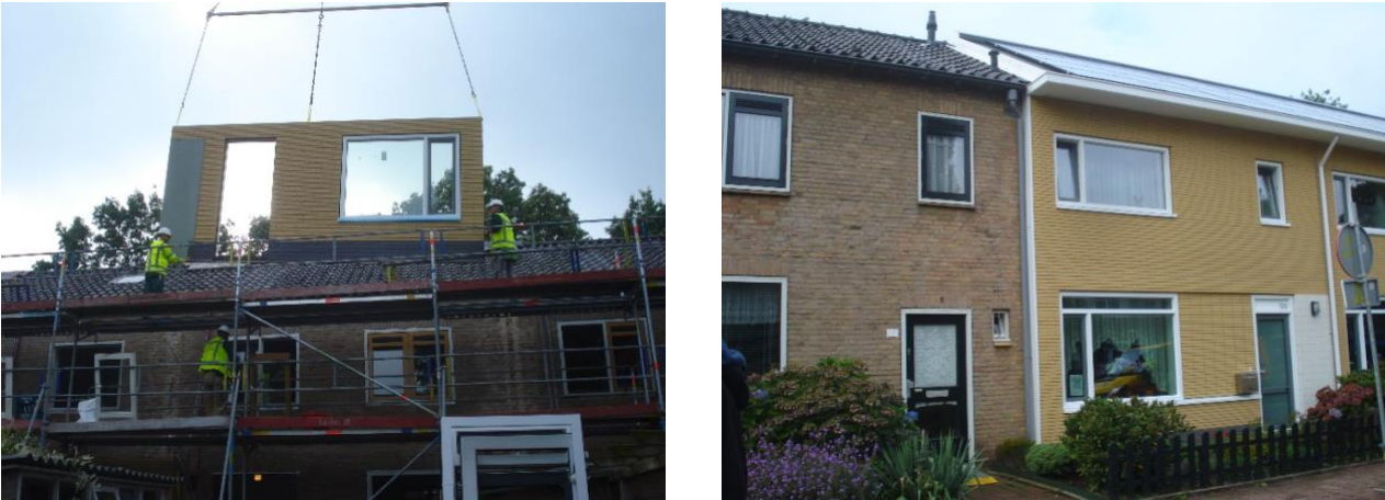
Figure 33 Prefab renovation with placing prefab elements on the existing façade (BAM)
